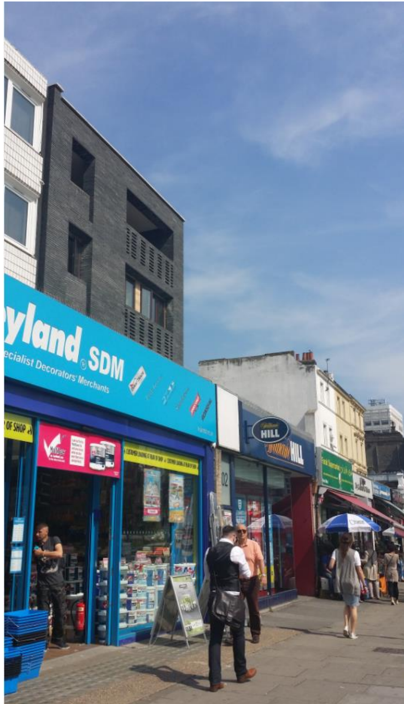
Front building of application site facing Edgware Road
